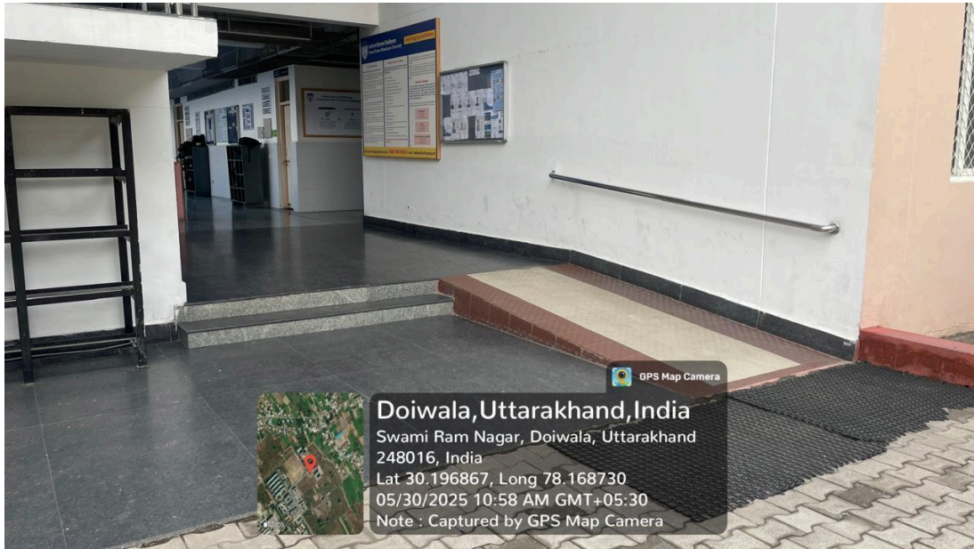
Ramp in School of Science & Technology, SRHU
